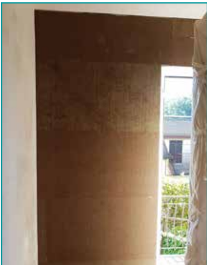
Nobilium® Thermalpanel laid on interior wall, without anchors, with layer of natural lime.
