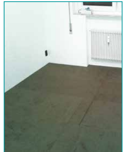
Nobilium® Thermalpanel for thermo-acoustic underfloor insulation.
